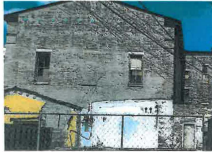
South Façade: (Rear)
