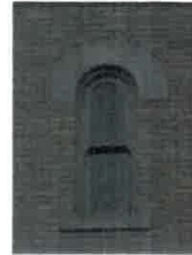
Third-floor accent arches
